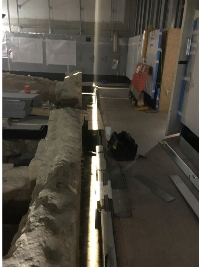
Architectural Lighting: Tillotson Design Associates Joseph / Local Projects / Foster + Partners
